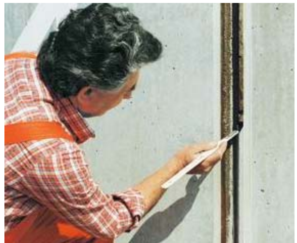
PCI Elastoprimer improves the bond of PCI joint sealants to the indicated substrates (see PCI primer chart).
