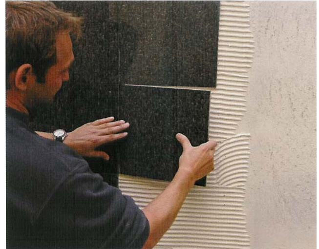
Laying of natural stone tiles on walls with PCI Carralight.
