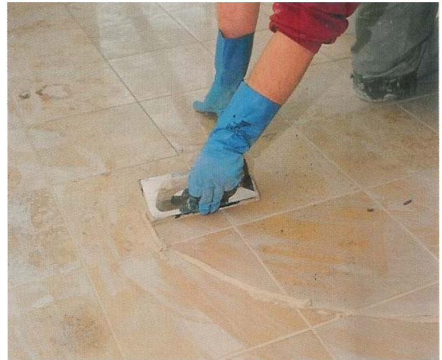
Even sensitive natural stone tiles can be securely laid with PCI Carrafug without staining.
